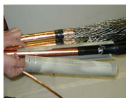
Removal of carrier
