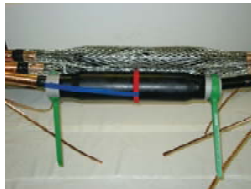
Joint body in position
